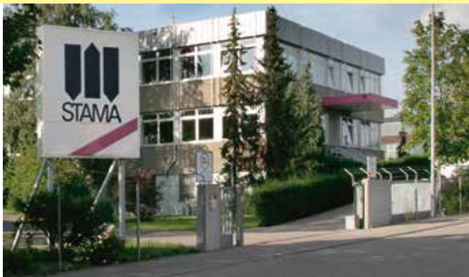
STAMA plant Schlierbach
